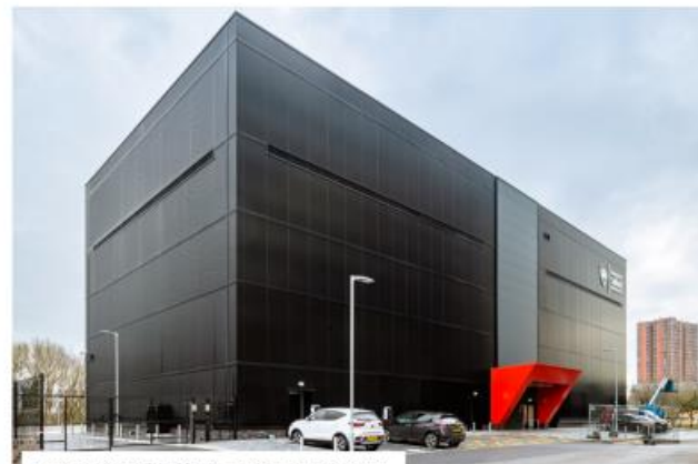
University of Salford - Energy House 2.0
