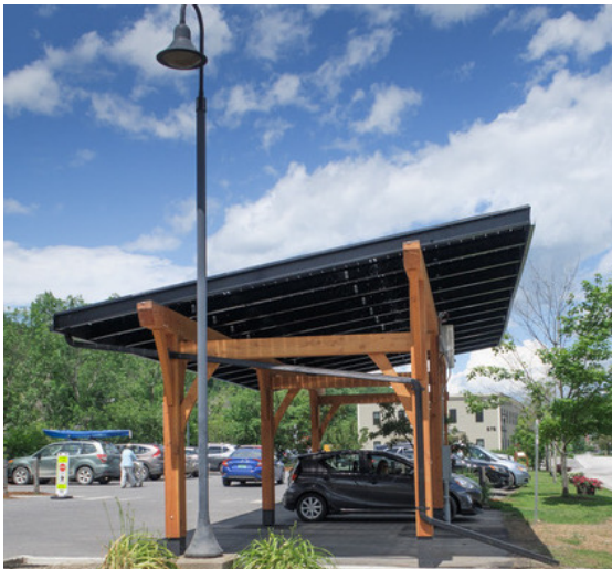
Example of Solar Canopy
