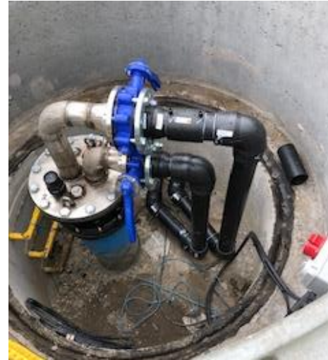
Geothermal wellhead with mine water pipe, in construction. BGS© UKRI
