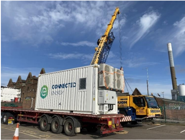
Batteries being craned into position
