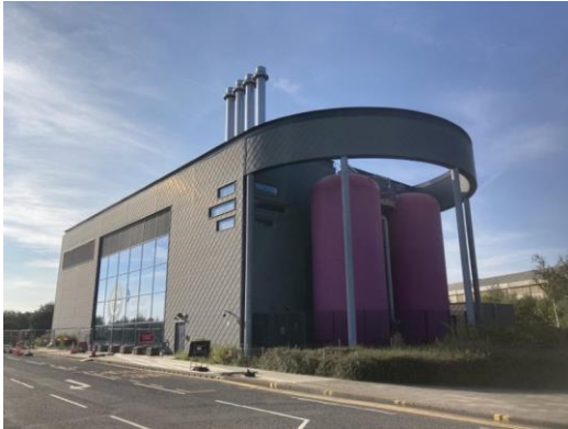
Existing CHP Energy Centre
