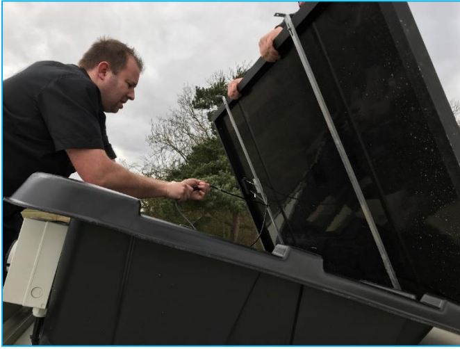
Installation of solar PV with Battery backup
