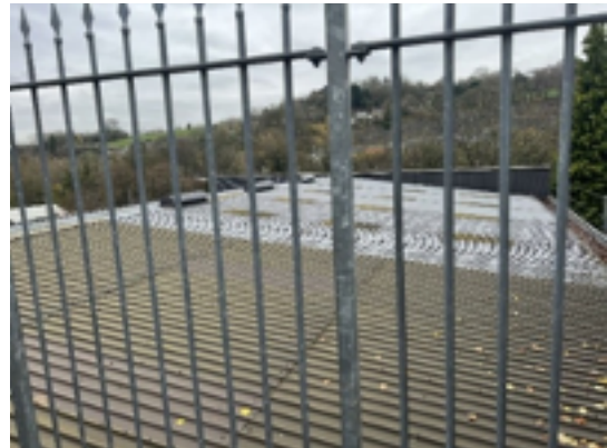
FIGURE 11-TWIGG STORES' EXTERNAL ROOF
