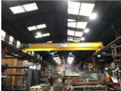
FIGURE 16 TWIGG STEELYARD INTERNAL ROOF STRUCTURE
