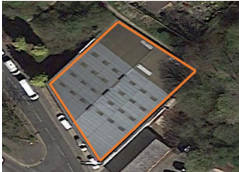
FIGURE 2 AERIAL VIEW OF THE TWIGG STORES SITE; SUITABLE ROOFING AREA OUTLINED IN WHITE
