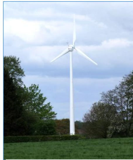
EO Cycle 25kW installed 2019 at Sandy Lane Farm, Shropshire
