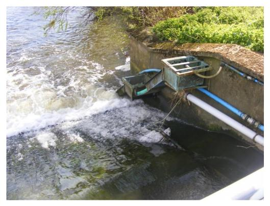
Figure 7. Eel pass on South side of weir.
