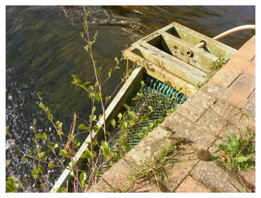
Figure 6. Eel pass on North side of weir.
