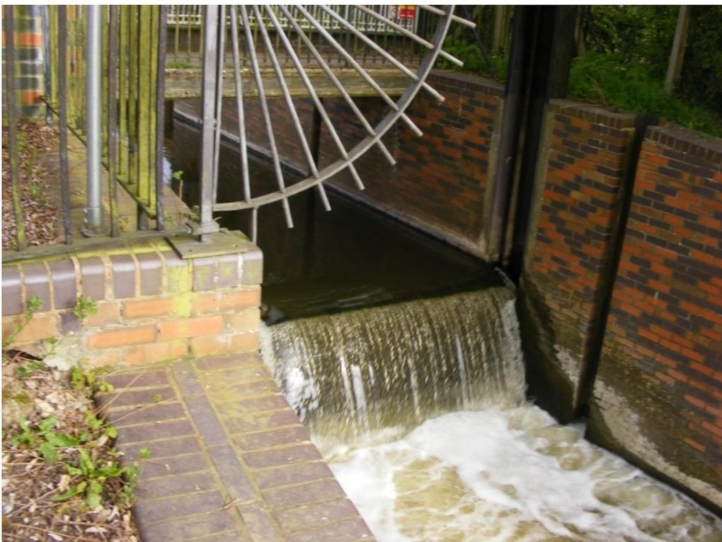
Figure 3. Single sluice.
