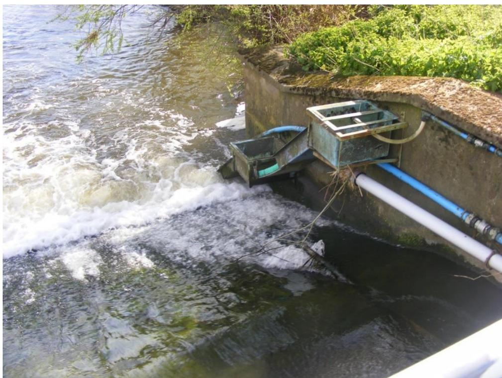
*Figure 7. Eel pass on South side of weir.*
