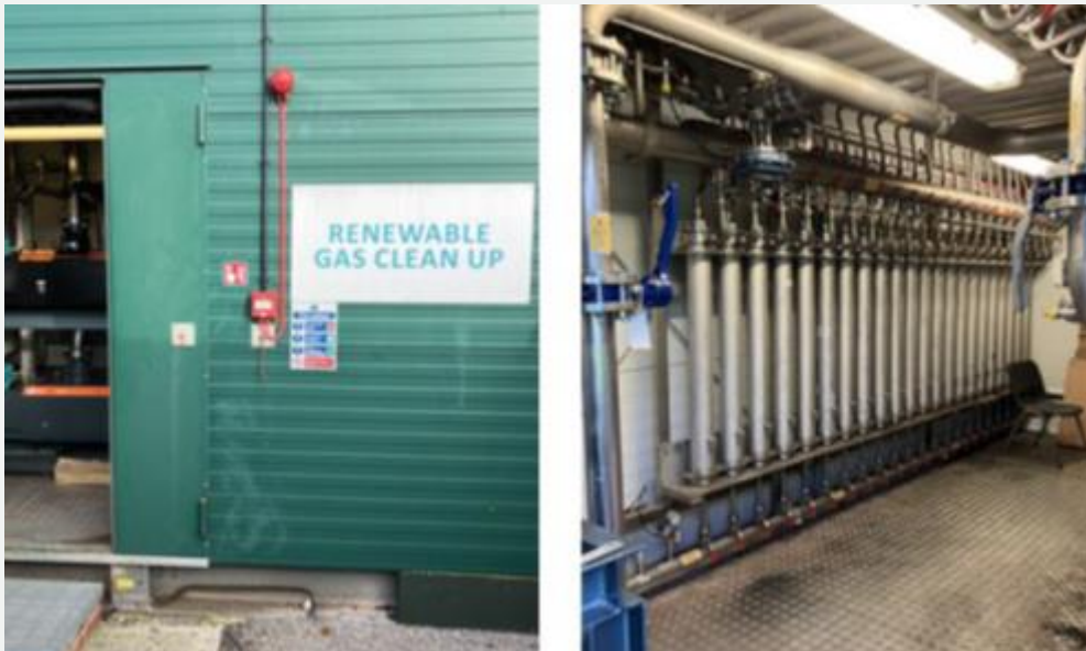
Figure 5 - Gas cleansing membranes converting raw biogas to biomethane
