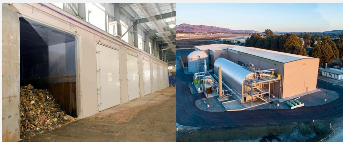
Figure 7 - Dry anaerobic digestion systems: (L) batch-based tunnel digester; and, (R) horizontal continuous plug-flow digester
