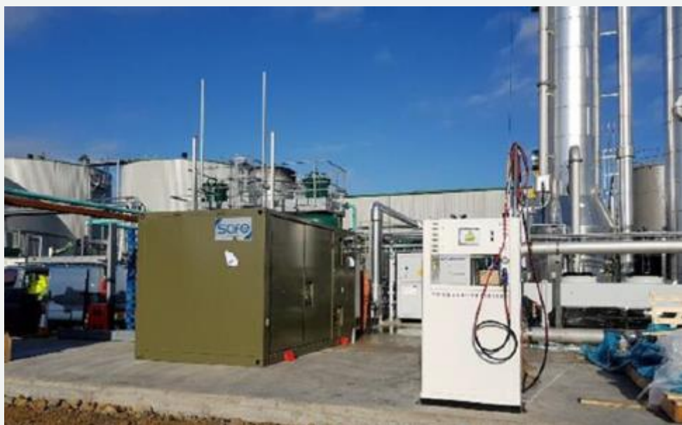
Figure 10 - Depot scale bio-CNG fuelling point
