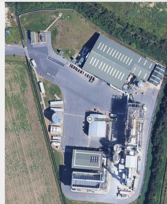
Biomass Building no #3
